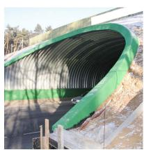
concrete headwall - bevelled end.
