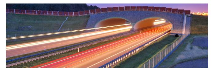
ViaCon ViaPlate & SuperCor® & UltraCor® are used mostly as buried flexible steel bridges & culverts, also called soil-steel structures. They are used for roads and railways infrastructure as well as for some industrial applications.
